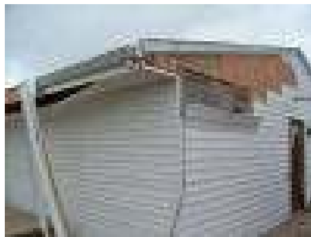
Shop SE side siding blown off.
